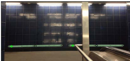
Fig. 4: Intersection 5 with green running lights moving to the left (movement was achieved by using GIF).
